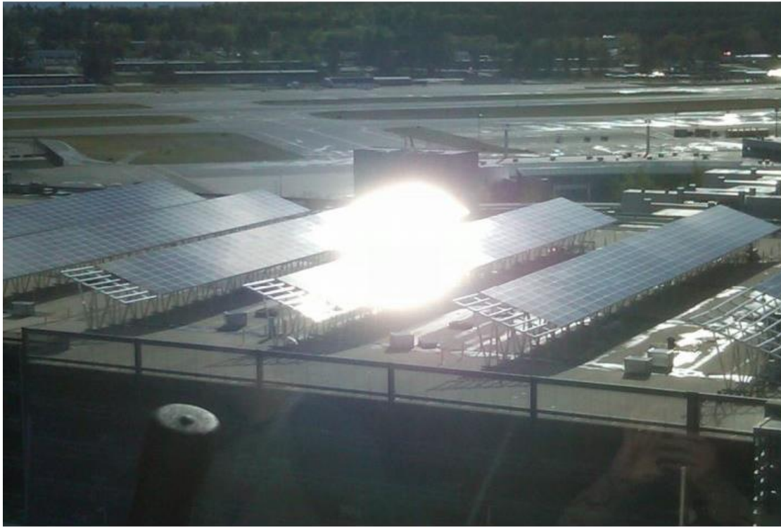
Plate 6 - Glare experienced in the Control Tower at Boston Regional Airport from an adjacent PV array
