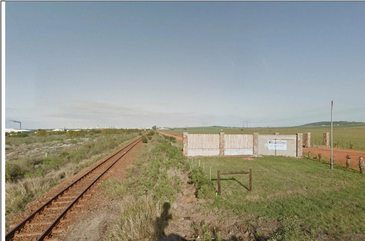
Plate 6, The railway running immediately north of existing Mossdustria
